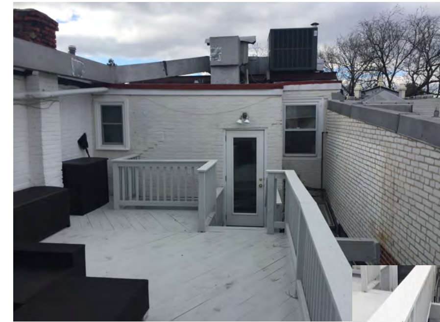
EXISTING 3RD FLOOR / DECK
